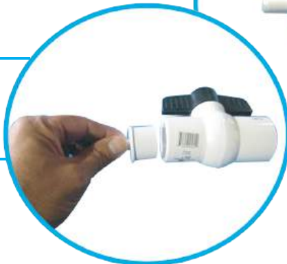
Glue the adapter into the 1" valve using PVC glue, then glue the valve into your water supply to control flow.
